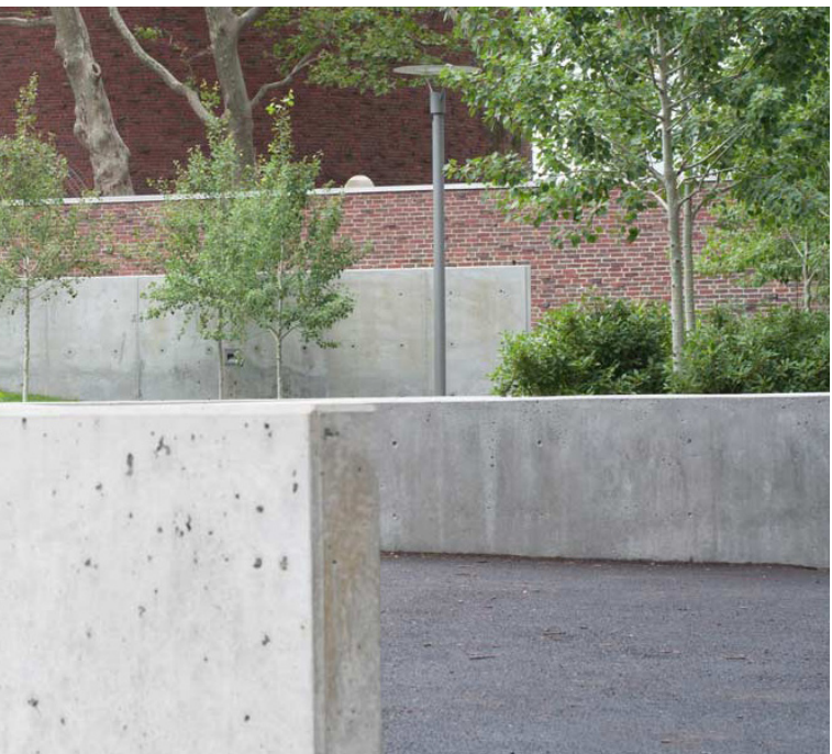
Off Form Concrete Walls
